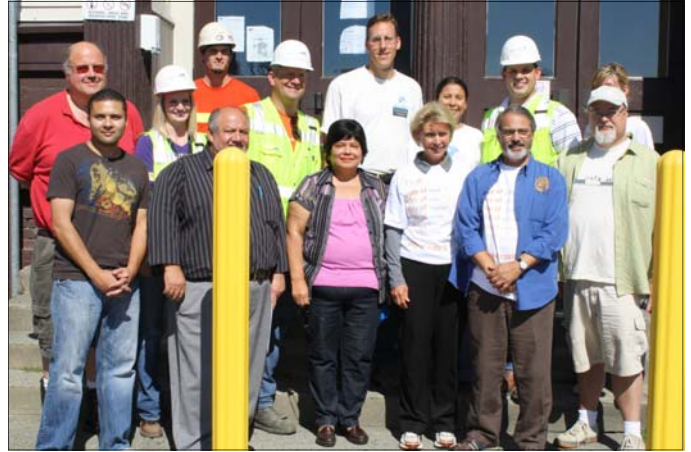
Through a project organized by United Way, new stairs are being built for the North, South, and West entrances of the El Centro building. Mil gracias to Mortenson Construction, Architects W/O Borders, Engineers W/O Borders, and McKinstry for their generous pro-bono efforts. The project will save El Centro de la Raza over $180,000 in necessary repairs.
